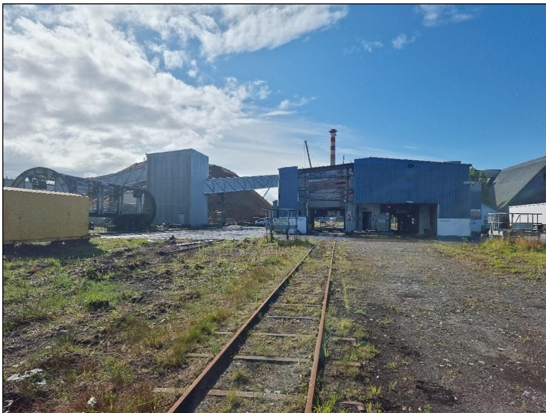
Plate 6-31 Edenderry Power Station (background) in the west of the site is classified as Buildings and artificial surfaces (BL3).
